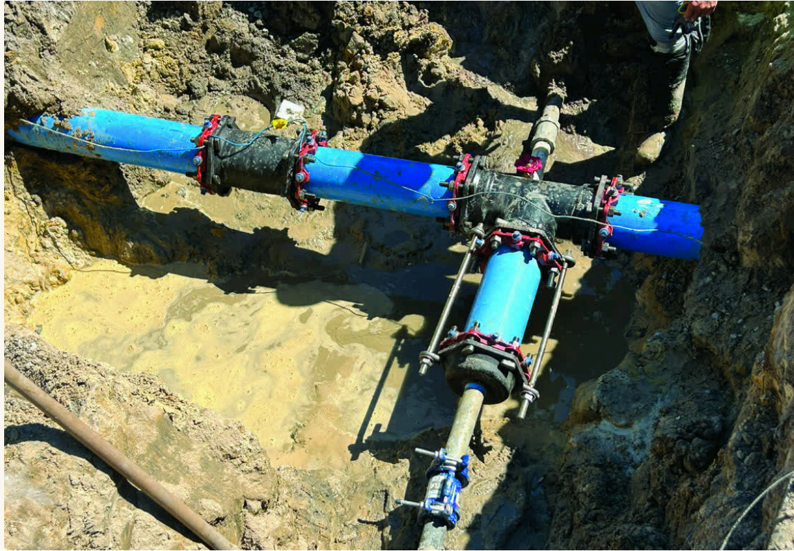
The new water main joined in the trench before the ground closes back over it. Courtesy Neel-Schaffer.
