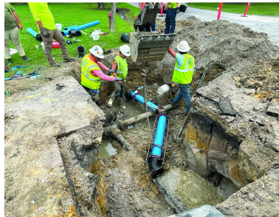
Crews on Kimberly Drive replace the old asbestos cement water line with new PVC main. Courtesy Neel-Schaffer.
