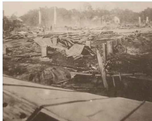
Collapsed roofs and bare chimneys where storefronts had stood.
