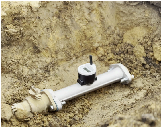
One of more than 4,700 new water meters installed across Moss Point, ending years of estimated bills. Photo by Experienced Results.
