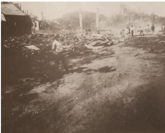
A resident walks through the debris the morning after.
